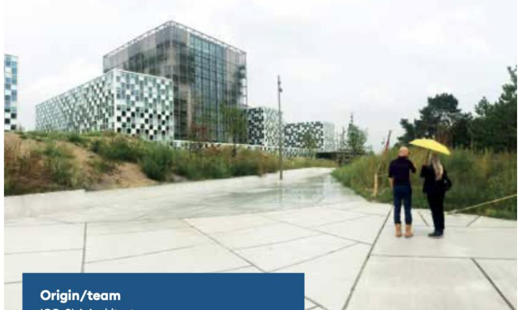
Photo: SLA Architects
